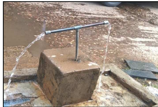
Manuguru ULB (Non-fixing of taps to the stand posts)
